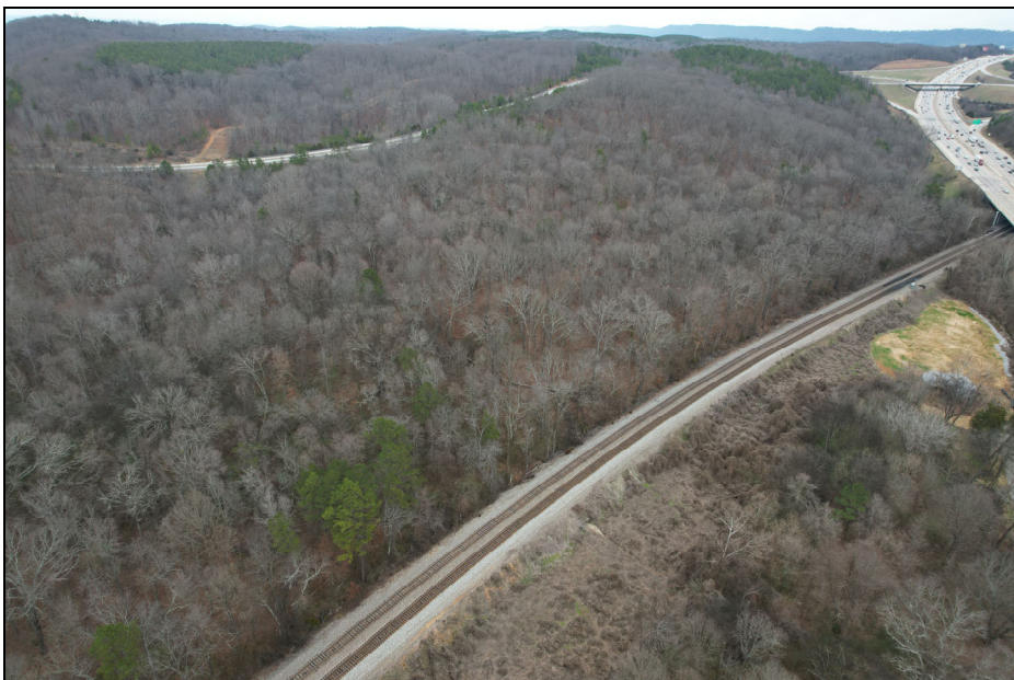
SOUTHWEST SIDE OF SUBJECT FACING NORTHEAST
