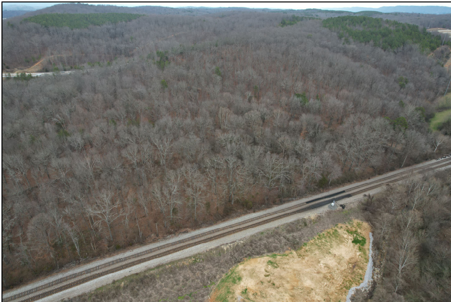
SOUTH SIDE OF SUBJECT FACING NORTH
