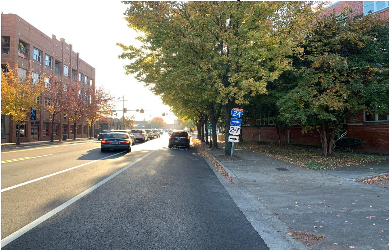
View from Cherokee Blvd Facing Southeast
