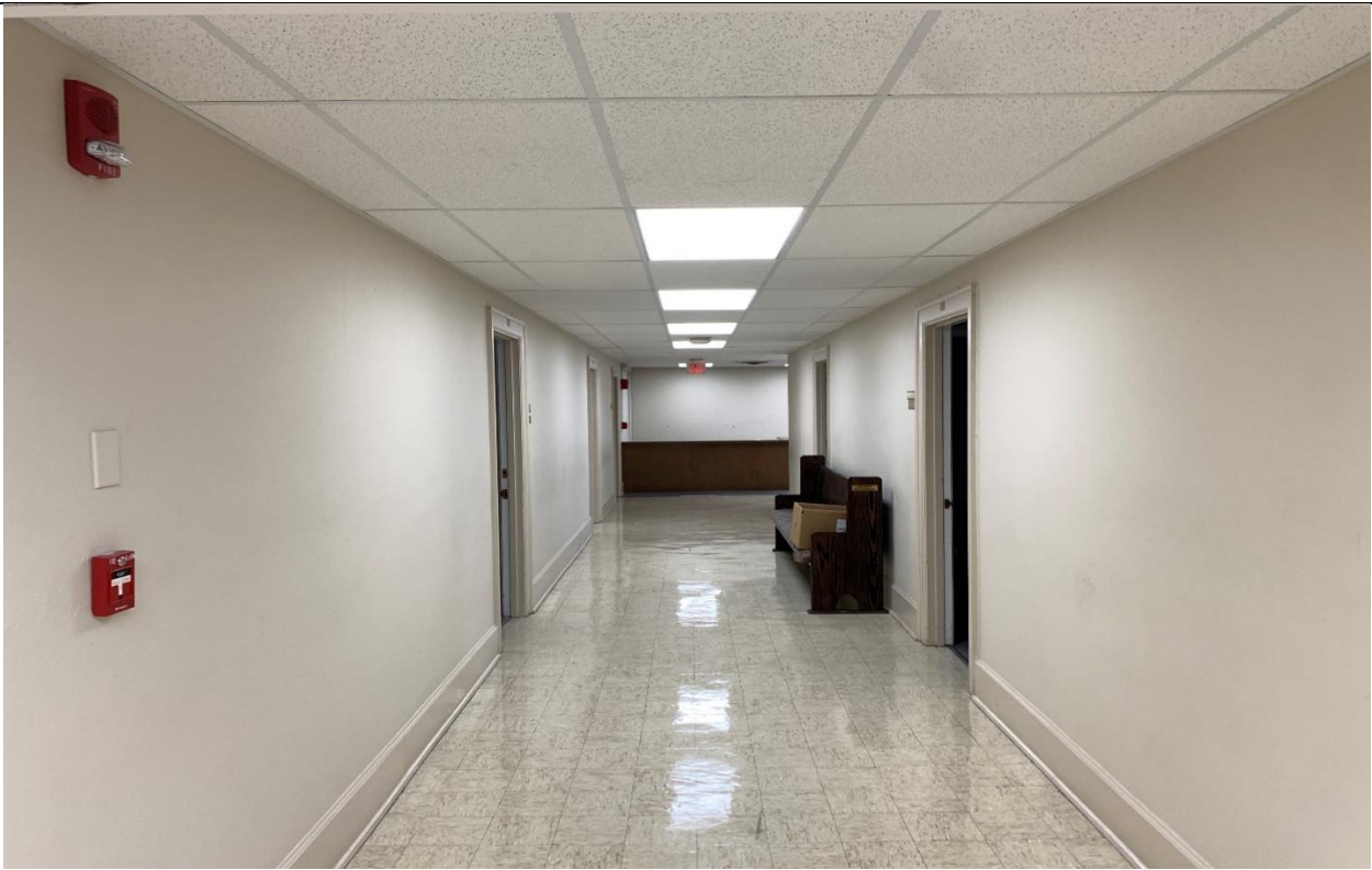
Typical Office Space – 2 nd Floor
