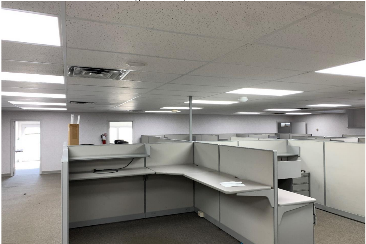
Typical Office Space – 4 th Floor
